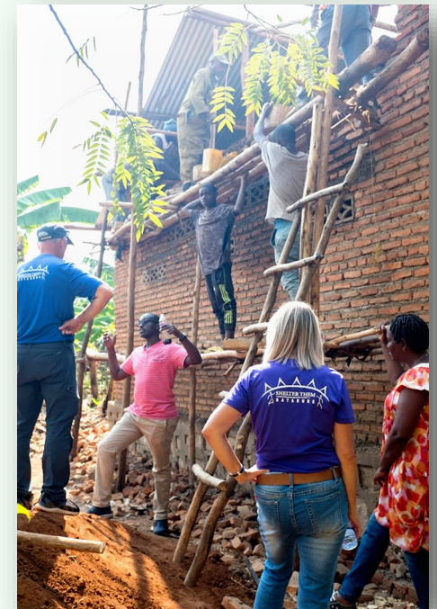
Construction of buildings in Gateko village
