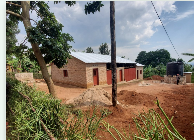
Drying Shelter System Facility
